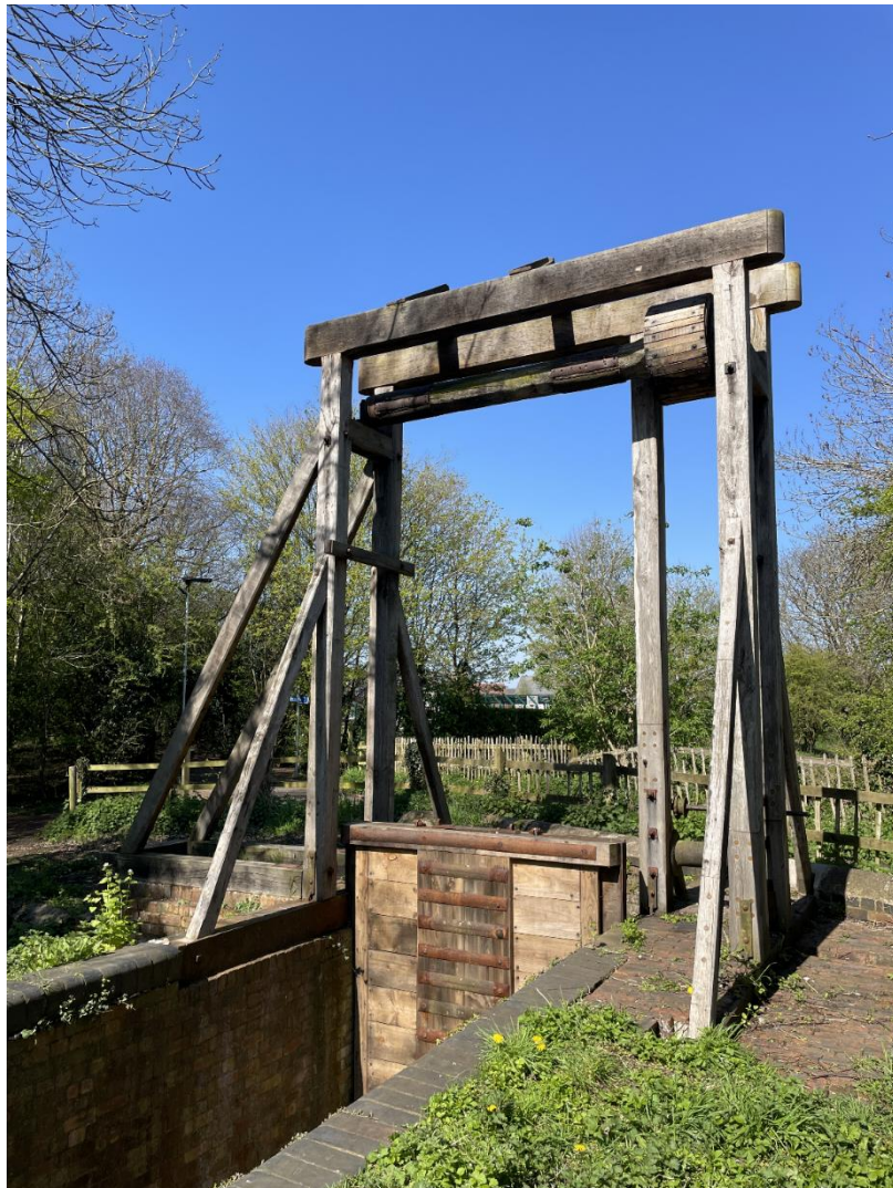
Figure 4: Enhancement of Grade II listed structures and public realm at Thomas Telford Hadley Locks
